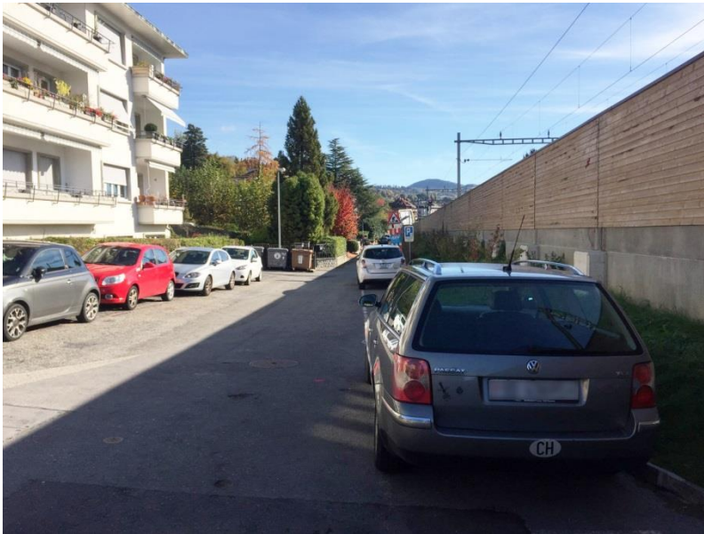
Ch. du Coteau 20, direction Pully
